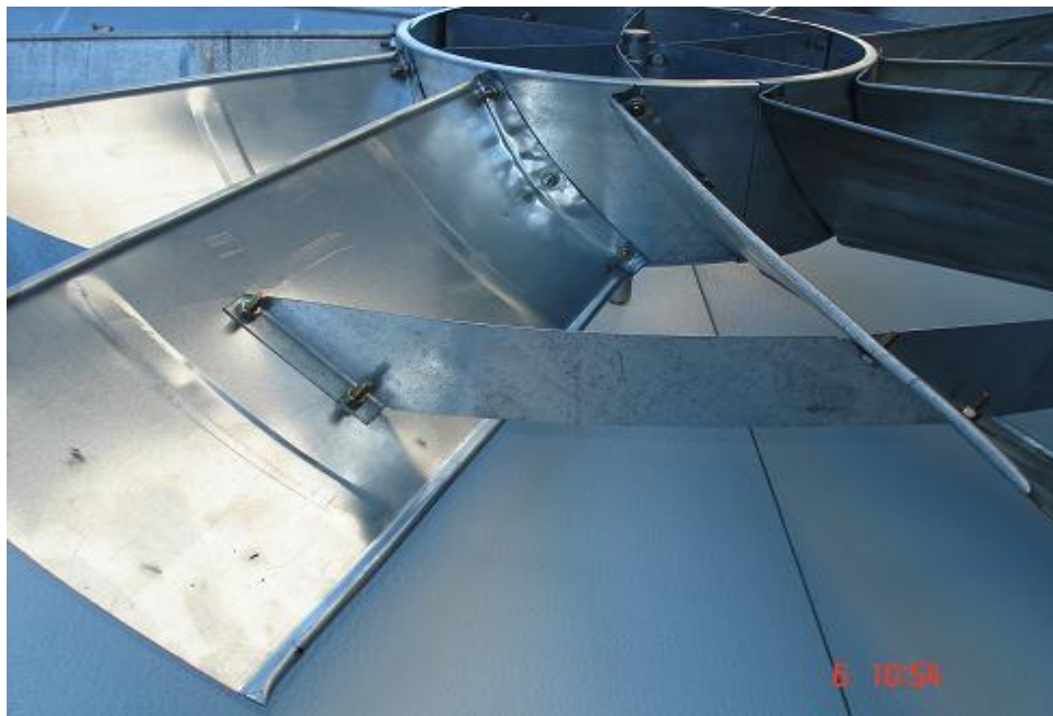
PHOTO 2 - SHOWS THE COMPLETED ASSEMBLY OF THE BLADE BRACES [BBR].
